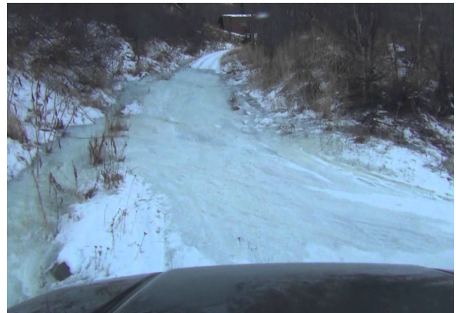
Improperly designed or maintained driveway that channels water onto the roadway.
